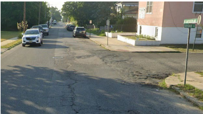
Bayview Avenue cerca de Broad Street
